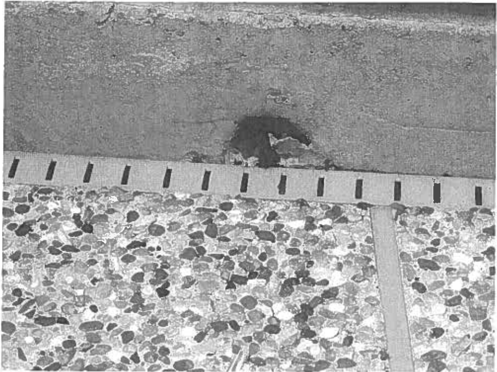
This is an exposed post-tension cable end and a Red Flag.
