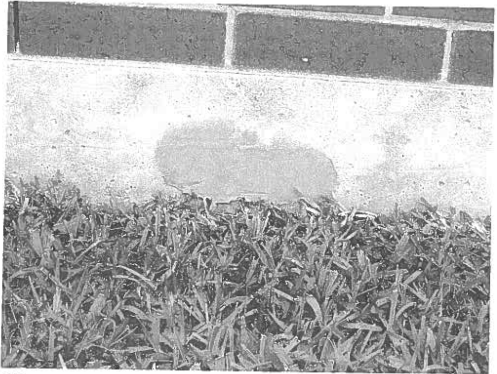
Figure 2.4 | Properly Covered Post-Tension Cable End
